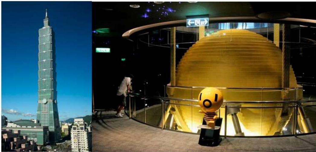
Figure 13: Taipei 101 skyscraper (left) and tuned absorber (right).
