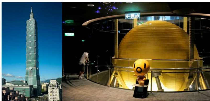
Figure 20: Taipei 101 (left) and tuned absorber (right)
